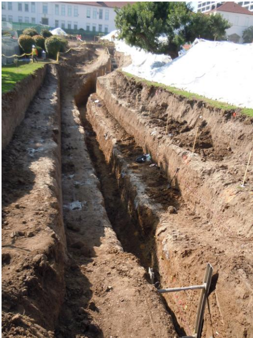
Figure 29: Leighton trench FT-2, excavated down the slope that was defined as the West Beverly Hills Lineament. This is one of five exploratory trenches excavated at the BHHS, part of which is seen at the top of the picture. Trenches were placed to cross and to expose the faults that were mapped by PB (2011) intersecting the BHHS. Despite the fault map (Figure 2), no faults were found in this trench.
