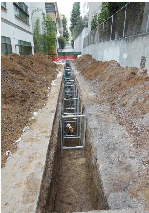
Figure 35: Leighton’s FT-5 trench excavation looking south down the center of the access driveway between the school (left) and the western property line (right). The trench was excavated to view an anomaly in the otherwise well-correlated older alluvial stratigraphy, and did reveal that the anomaly was caused by a fault, probably the fault shown on Figure 28 as “Holocene Activity Uncertain.” The geologic log of the trench is shown on Figure 36.
