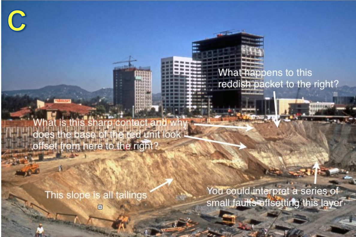
Figure 44 a-c: Three photos (a-c from top to bottom) reprinted from 35mm slides taken at an indeterminate time during building foundation construction at a site immediately south of the Constellation site, and used in support of the geological conclusion that there are no faults through the Constellation station site. The KGS faults, assuming their orientation was accurate, would appear under the foremost drill rig in the second picture and under the loader in the third picture, passing through a part of the excavation that is totally covered by a retaining wall. The first picture is looking at the excavation corner furthest from the mapped KGS fault location, more than 1,000 feet away. Only a scant percentage of the excavation is exposed well enough to provide any information. These photos are totally inconclusive to support any conclusion regarding the presence or absence of faults.
