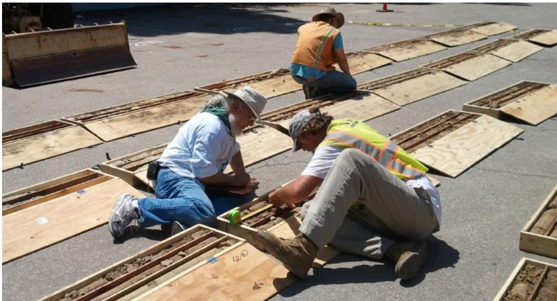
Figure 40: Parking lot side-by-side core comparisons were ultimately conducted to include every core taken by Leighton and many of the MTA cores. Reviews were conducted by full peer team of BHHS consultants, plus CGS and City of Beverly Hills as regulators, and also included AMEC representatives (who took the core samples for MTA). MTA boring logs were corrected and amended to reflect group observations. Visible team members are from CGS and Leighton.
