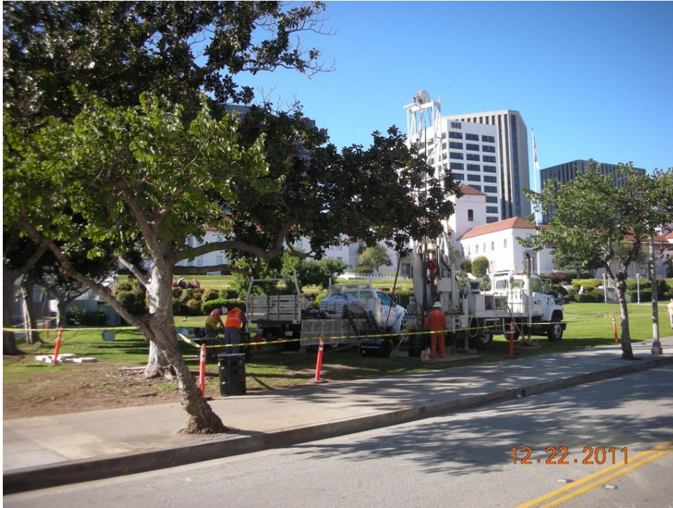
Figure 4: Fault investigation drilling begins at Beverly Hills High School. Several of the Century City high rise buildings in background are on top of faults mapped by MTA.
